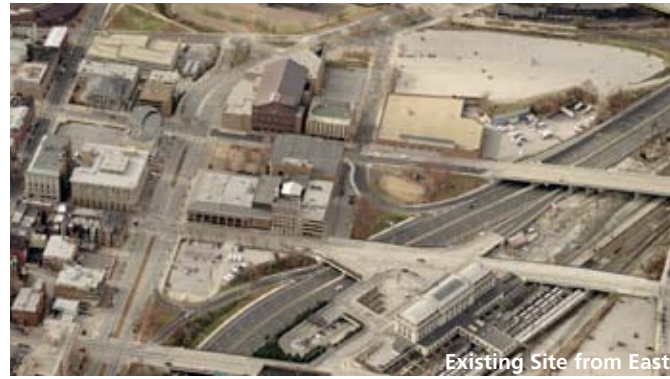
Existing Site from East
